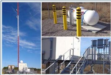
The Coast Guard installed radio antennas, a propane-powered generator and computer equipment to add Rescue 21 capabilities to an existing Navy tower near the Pamlico Sound in North Carolina. U.S. Coast Guard photos.
