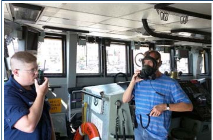
Allen Balough, a lead engineer for the C4ISR program (right), tests the new interior communications system with a Coast Guard Cutter Spencer crewmember after installation of leaky coax cable. The installation took place in Boston July 18-21. U.S. Coast Guard photo.
