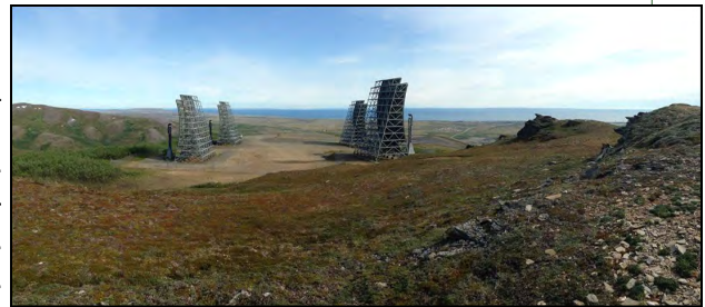
The old Cold War Troposcatter antennas still stand at the White Alice facility right outside of Nome.
