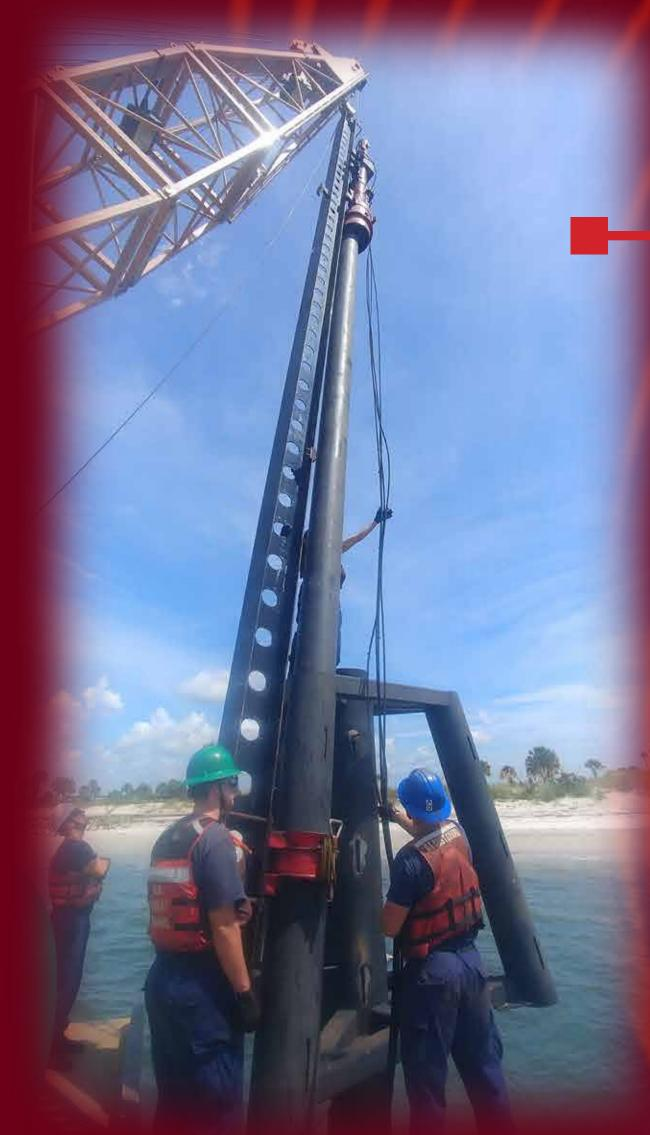
The WLIC's single-piston diesel hammer has the ability to punch pilings at an angle, as needed on ice structures like this one on the James River.
