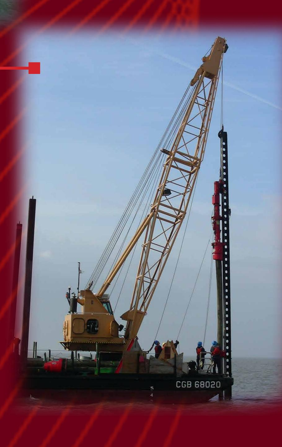
Crewmembers finish a single-pile wood structure, which serves as an ATON for commercial traffic to enter busy ports.
