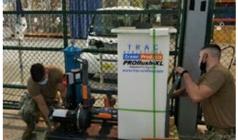
PATFORSWA Engineers unbox flushing unit.
