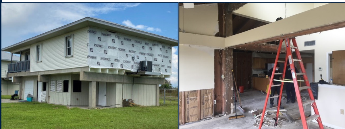
Extensive interior and exterior repairs were made to the Unaccompanied Personnel Housing and family housing units following Hurricane Ida.
