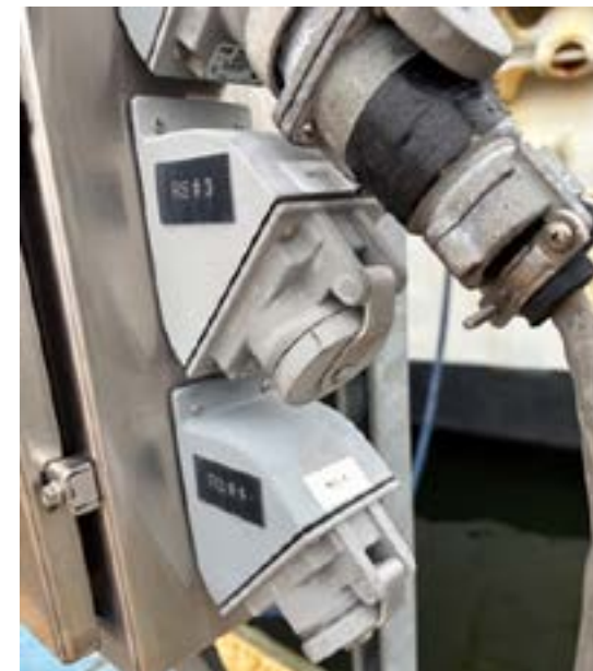
Example of a cracked telecom cover cap on the pier at Base Portsmouth
