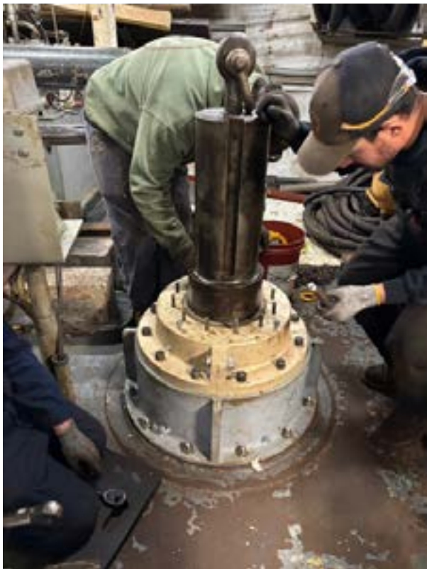
Upper bearing renewed/installed
