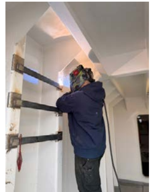
DCs installing brackets to CGC Storis
