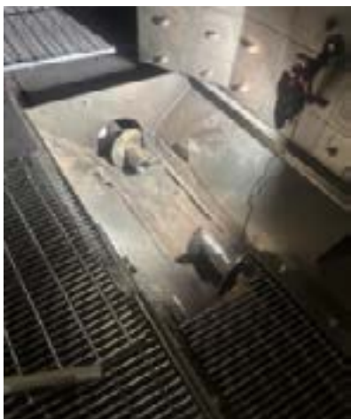
Removed Damaged shaft/bearing
