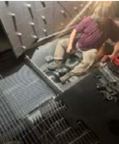
Removing damaged parts
