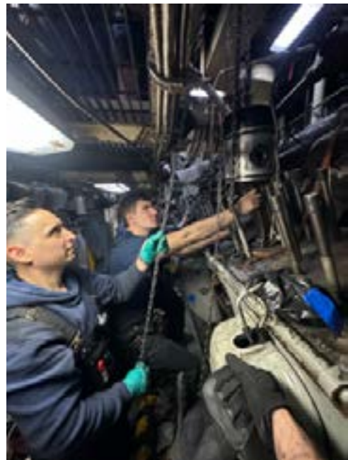
Removing damaged parts
