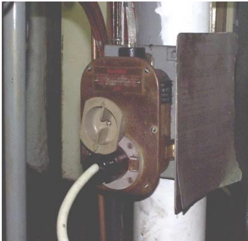
FIGURE B-1 – 450 VAC SWITCHED RECEPTACLE OUTLET
