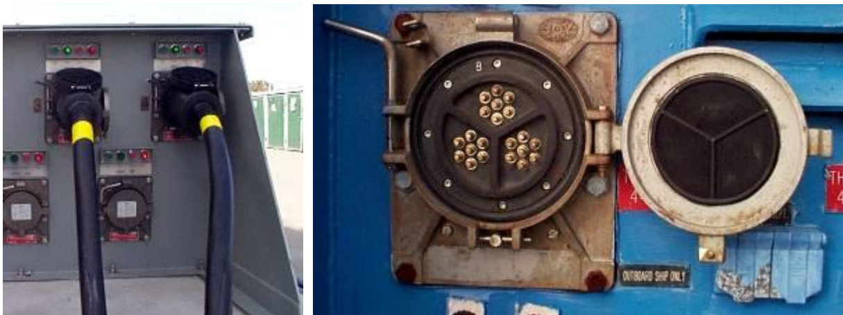
FIGURE A-2 – MIL-C-24368/2 SHORE POWER RECEPTACLES
