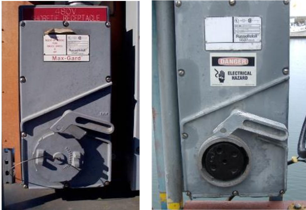
FIGURE A3 – RUSSELLSTOLL MAX-GARD® DBRS2404 RECEPTACLE WITH INTERLOCKING DISCONNECT SWITCH
