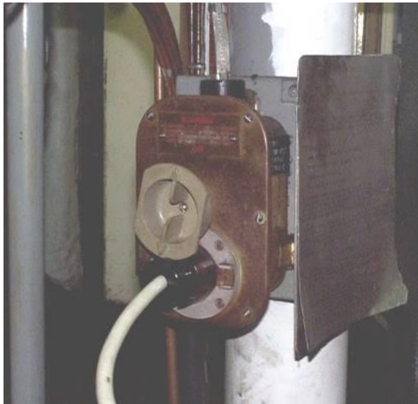
FIGURE B-1 – 450 VAC SWITCHED RECEPTACLE OUTLET
