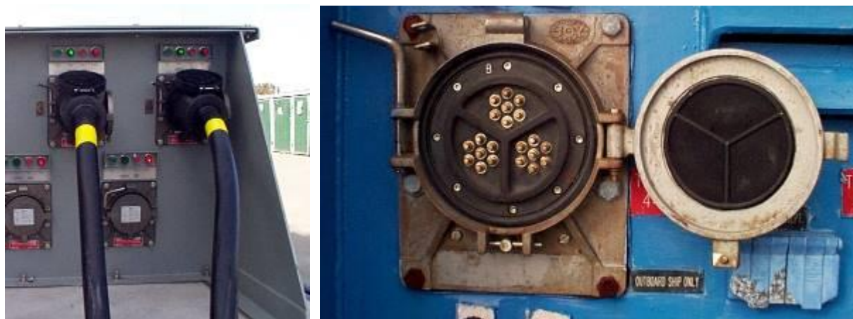
FIGURE A2 – MIL-C-24368B/2 SHORE POWER RECEPTACLES
