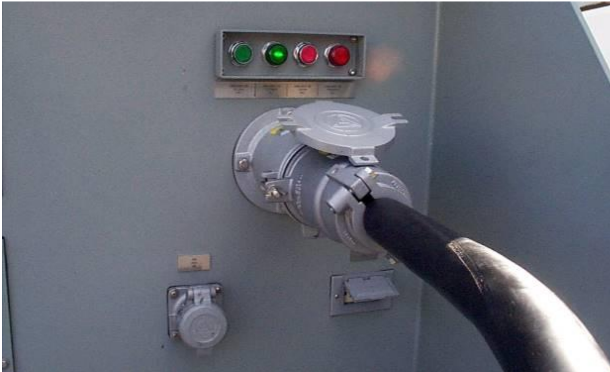
FIGURE A1 – TYPICAL SLEEVE AND PIN RECEPTACLE FOR SHIP REPAIR CONTRACTOR USE
