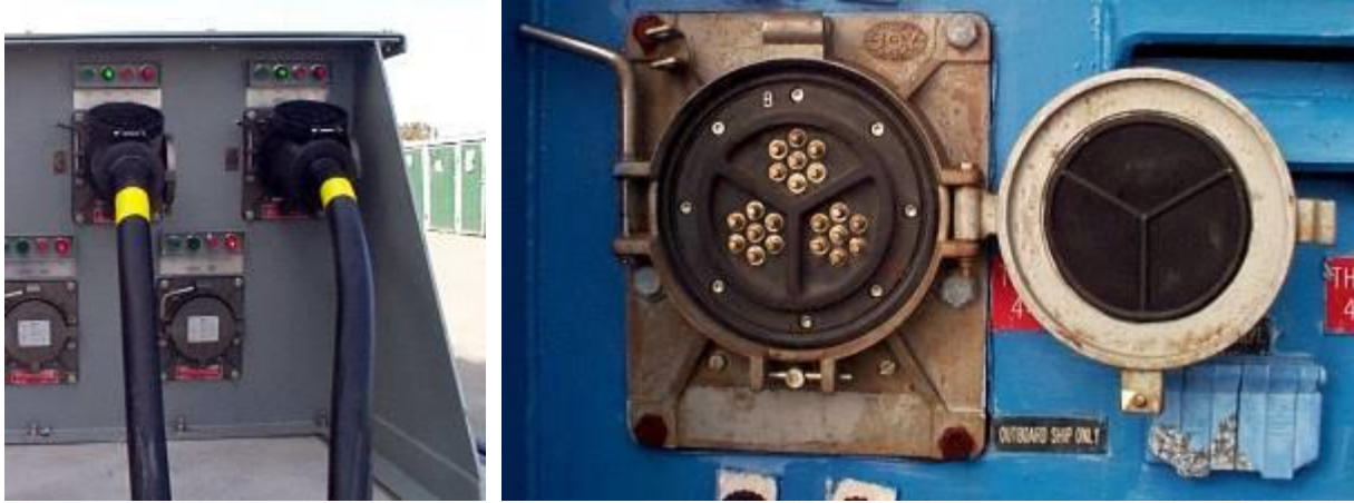
FIGURE A2 – MIL-C-24368B/2 SHORE POWER RECEPTACLES
