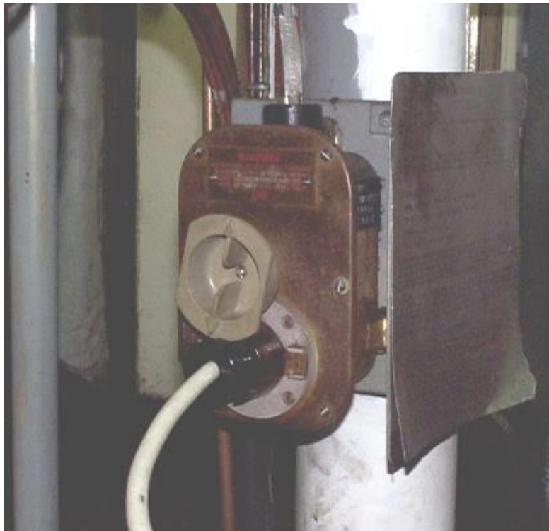
FIGURE B-1 – 450 VAC SWITCHED RECEPTACLE OUTLET
