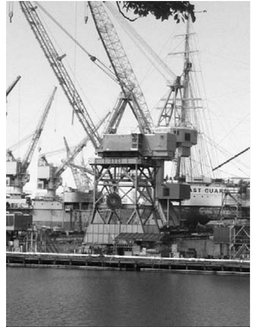
Electricity powered Tower Crane #5 with the Coast Guard Cutter EAGLE in the background.
