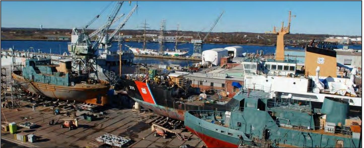
A snapshot of the Coast Guard's In-Service Vessel Sustainment (ISVS) Project throughout 2015 is featured with four ISVS cutters on the Yard's waterfront. Left to right on the shiplift are: 140' BRISTOL BAY; 225' OAK; 140' PENOBSCOT BAY. Barque EAGLE is pictured pier side in the background (center). The Yard com-
