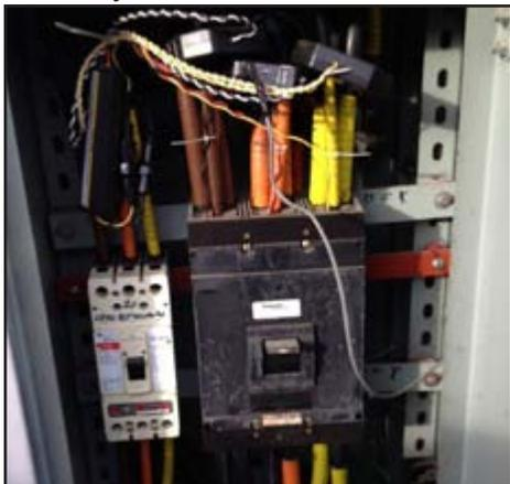
*The meter for Buildings #3 & #31 (pictured at left) is was one of 96 meters mounted in various Yard facilities and shore ties, providing critical energy data for the project.*
