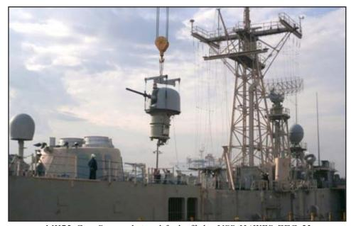
MK75 Gun System being lifted off the USS HAWES FFG-53
