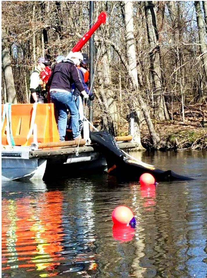
A 25-foot section of inland underwater oil barrier is laid out on a dock prior to deployment, April 23, 2018, in Kalamazoo, Michigan. The three-foot-high barrier is made of PVC and X-Tex fabric, and is designed to let water flow through while trapping oil. Weighted chains and scour flaps prevent oil and sediment from flowing underneath the barrier.
