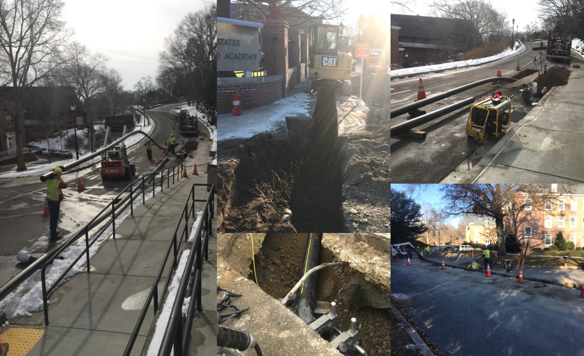
Natural gas line installation through main gate, down Tampa Drive and Harriet Lane.
