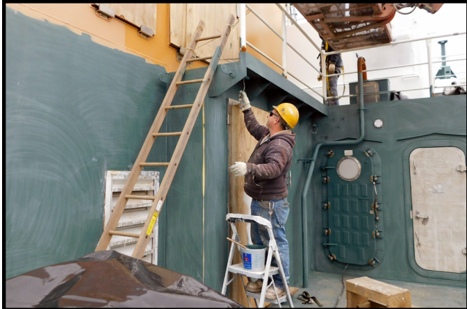
Yard Paint Shop employees finish up the primer coat on USCGC Fir’s 02 level superstructure.
