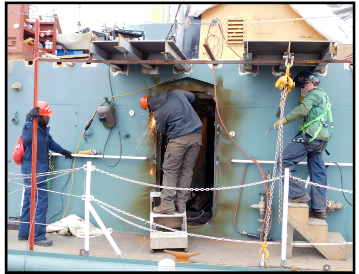
Welders aboard USCGC Mobile Bay perform repairs to deck stiffeners, which are installed to support boat davits. A contracted fire-watch keeps an eye on safety during the operation.
